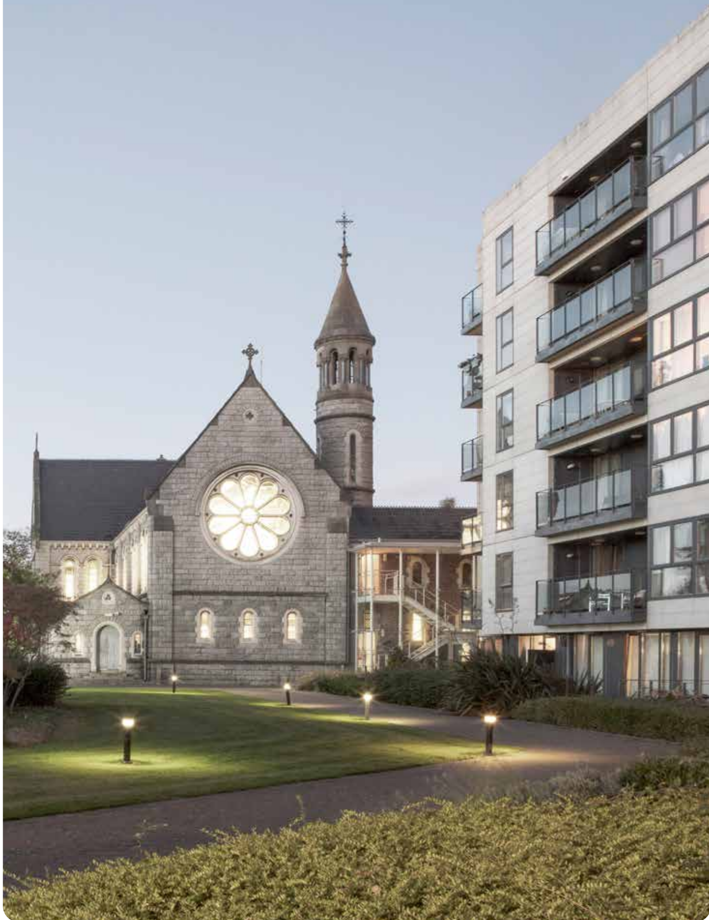
Figure 2: Higher density development with increased building height in a sensitive location at Mount Saint Annes, Dublin.
