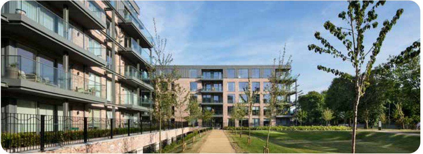
Figure 13: Increased building heights scaled and oriented to provide supervision of a public open space at Marianella, Dublin.
