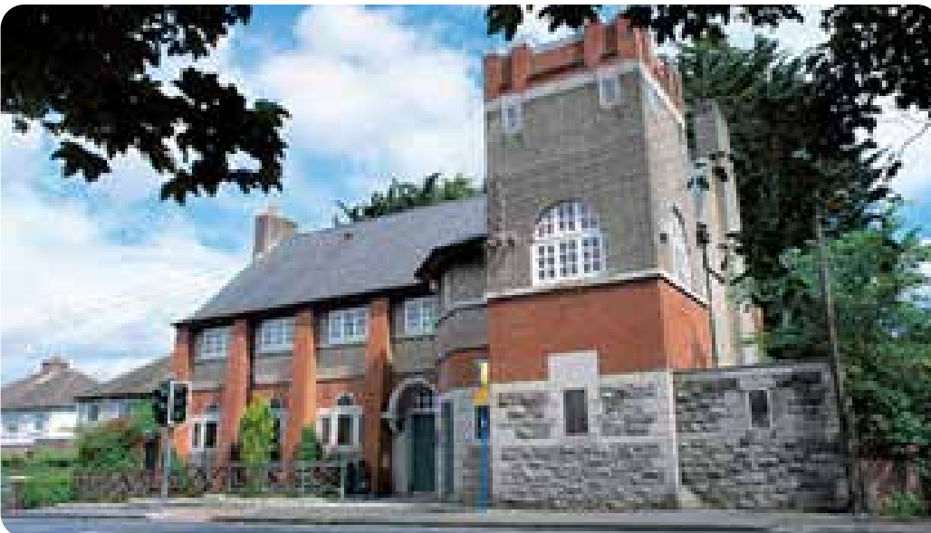
Figure 10: The Carnegie Library on Monastery Road in Clondalkin functions as a Local Marker. This function is achieved without a significant increase in building height but instead by the articulation of secondary mass perpendicular to the main building and its vertical expression as a tower.
