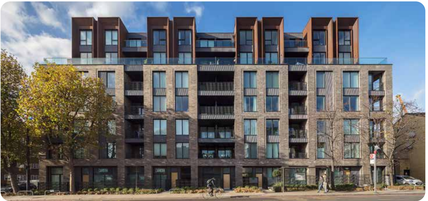
Figure 6: Development at Camden Courtyards, London where the apparent height of the building has been reduced by setting back the top two floors.
