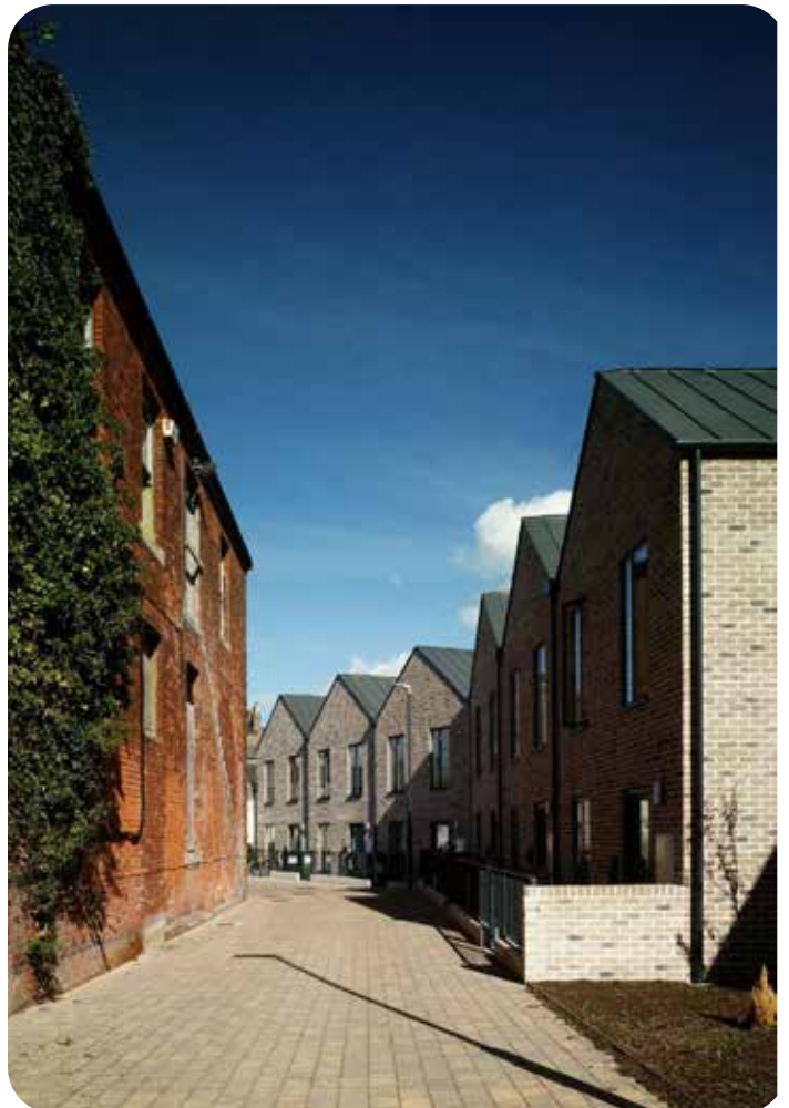
Figure 49: The twelve dwellings at St. George's Place, Dublin provide high quality energy efficient A1 rated dwellings with front and rear garden space that are suitable for families. A higher density of 67 dwellings per hectare maintains own door entry and a low-rise form of development.
