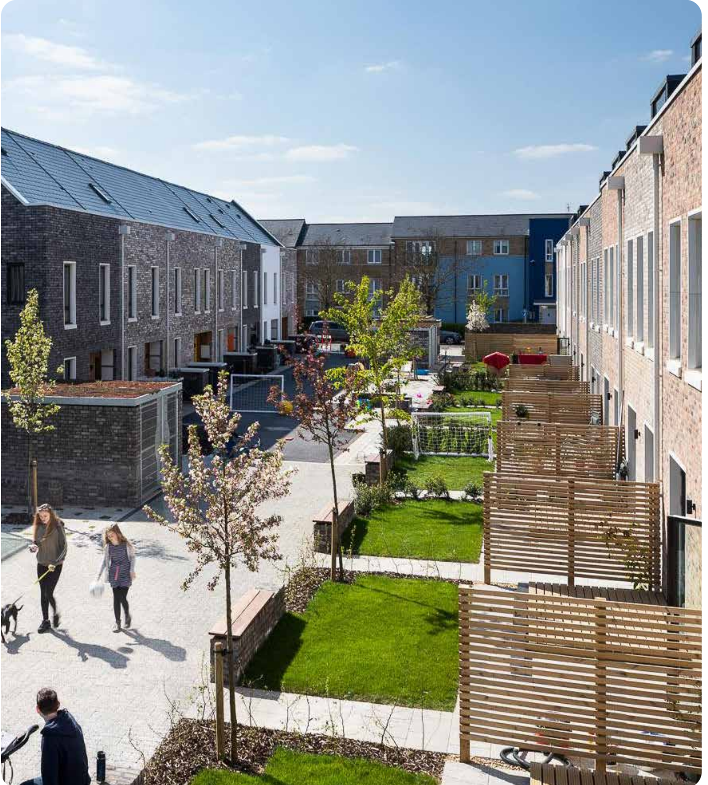
Figure 22: The development at Marmalade Lane achieves higher densities at a predominately two-storey scale without recourse to increased building heights beyond the limited use of three-storeys.
